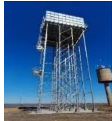
Upgrading of Orangeville WTW and Construction of Pressure Tower
