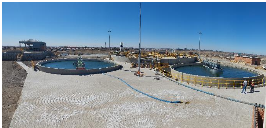
Upgrade of Refenggotso (Deneysville) WWTW Construction completed and the process of commissioning has been done
